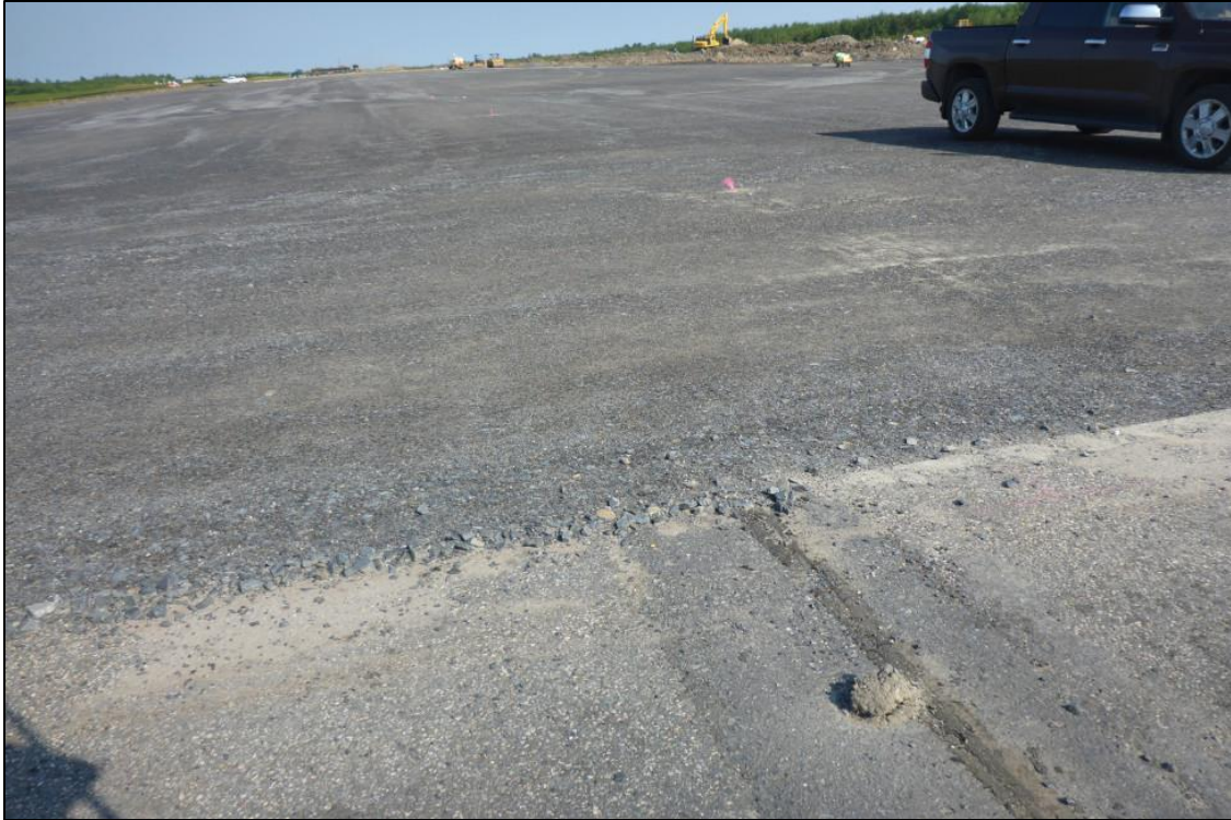
INL RY1331 009 (PCI = 100) (under construction)
