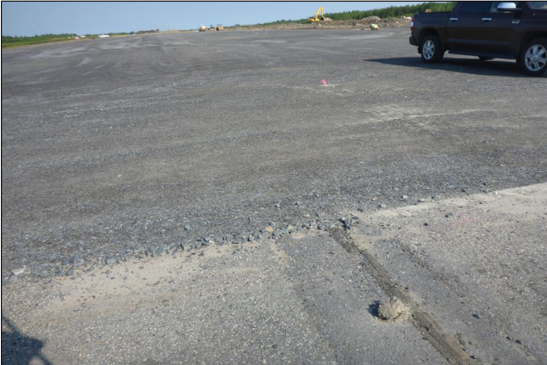
INL RY1331 008 (PCI = 100) (under construction)
