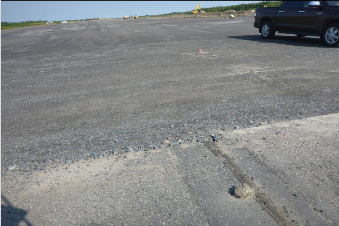
INL RY1331 007 (PCI = 100) (under construction)
